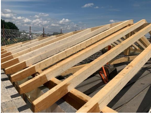
Main structure and secondary structure with wooden trusses, beams and purlins
