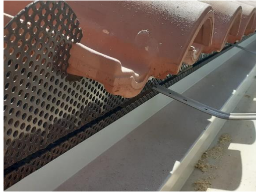
Installation of tiles following producers' instructions for optimal ventilation
