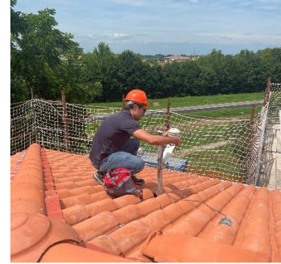
Installation of probes for the roof thermal performance monitoring
