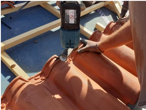
Installation of tiles following producers' instructions for optimal ventilation
